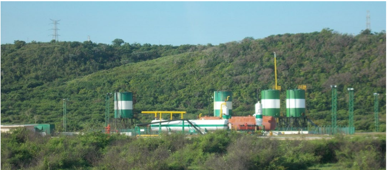
Figure 4: Ground level view of Santa Cruz oil field operation
