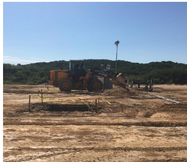
Figure 8 - Site prep for Alameda-3
