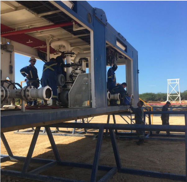
Figure 5 - Rig set up for Alameda-3
