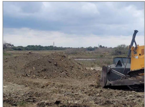
Amistad-2 well-pad earthworks continuing.
