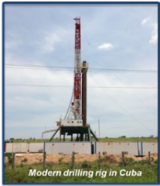
Modern drilling rig in Cuba
