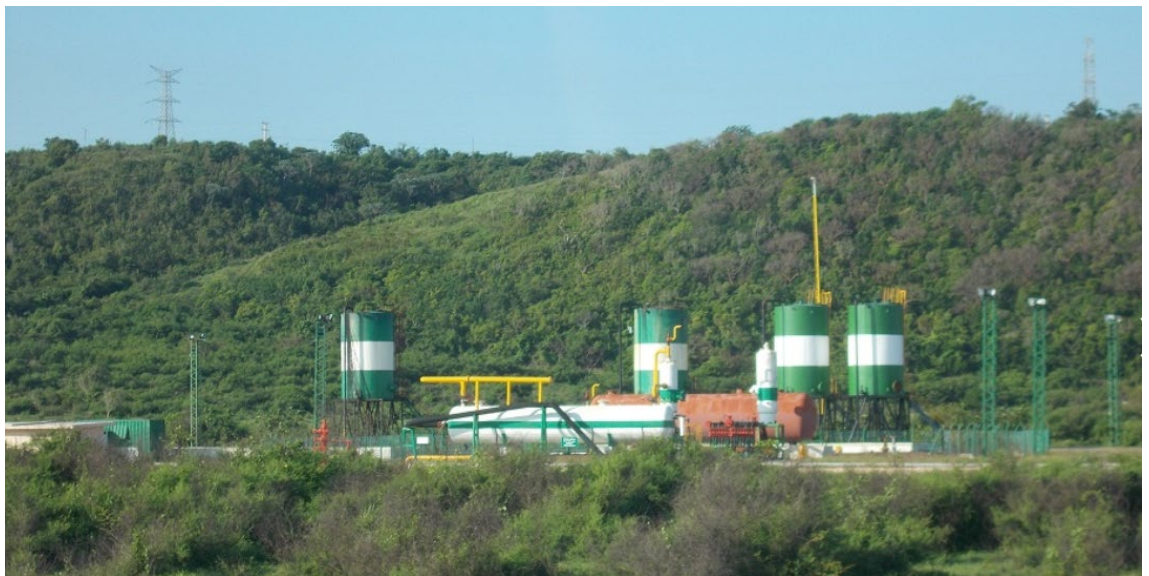
Figure 4. Ground level view of Santa Cruz oil field operation
