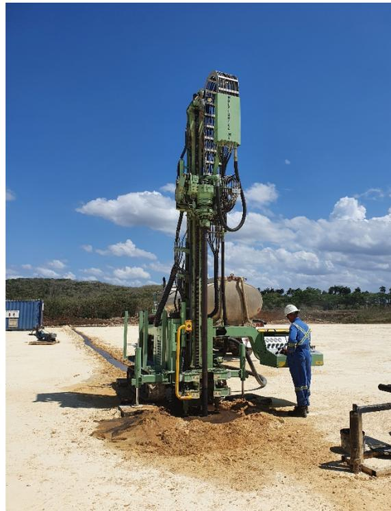
Figure 2 - Geotechnical test well at rig location
