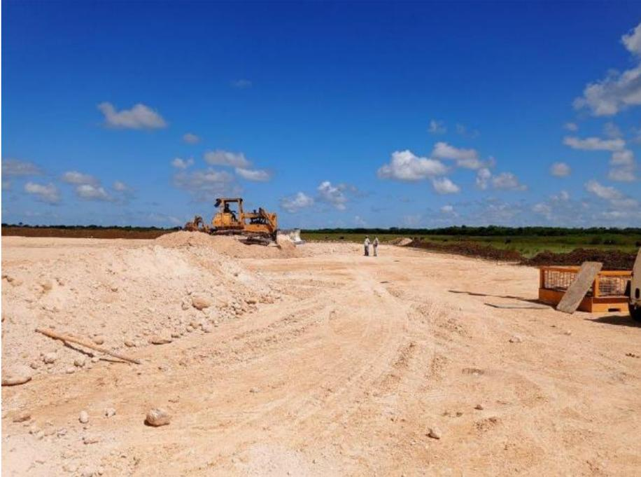
*Figure 2 - Zapato-1 well pad now building up the second tier*
