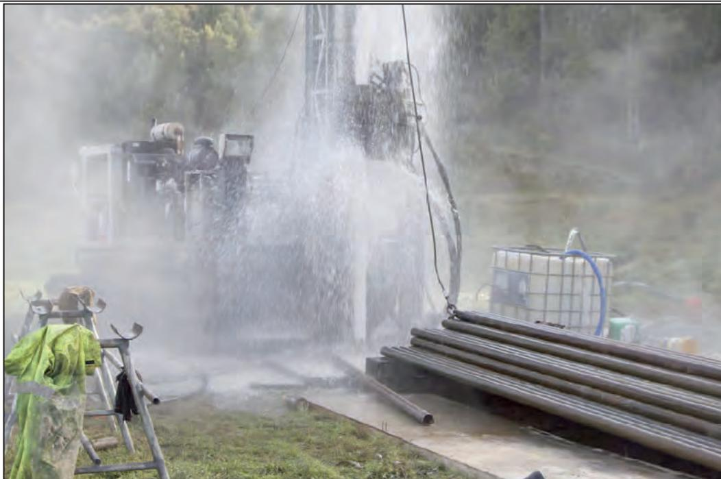
**Figure 2-7:** Artesian flow from the Cobden Limestone (Kotuku-1a) indicates high reservoir pressures occur in compartments in the formation
