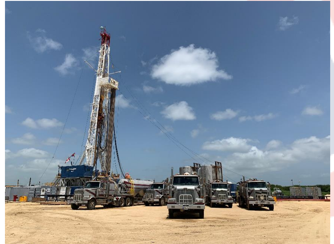
Casing on bottom - 15 July 2023
