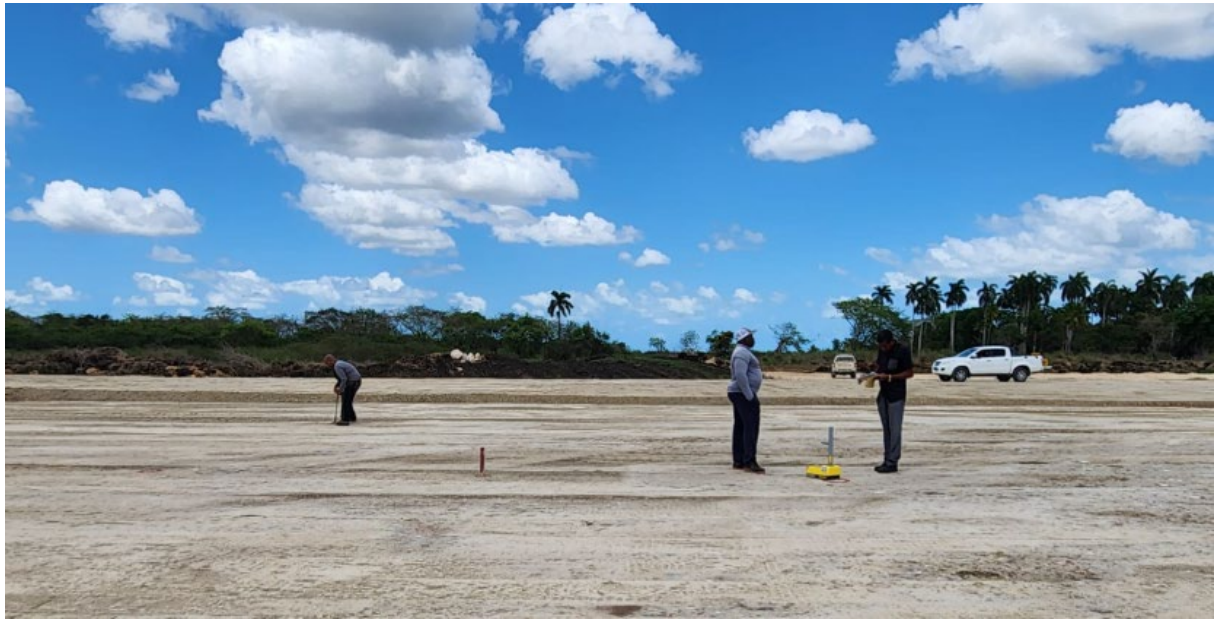
Figure 5 - Compaction and levels testing at Pad 4
