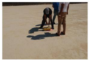
Figure 3 – Compaction testing of Alameda well pad
