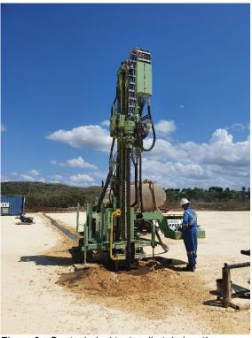
Figure 2 - Geotechnical test well at rig location
