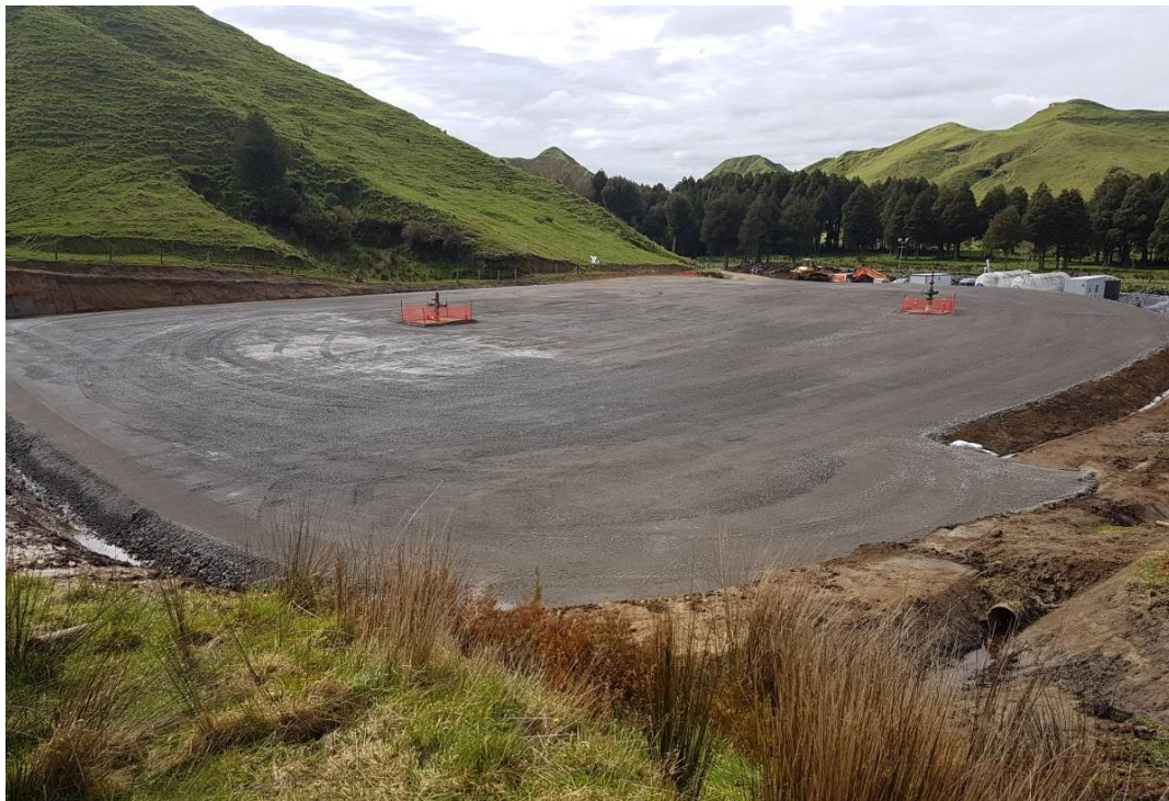
Completed Pukatea drilling pad with existing Puka-1 and Puka-2 suspended wells protection zones visible
