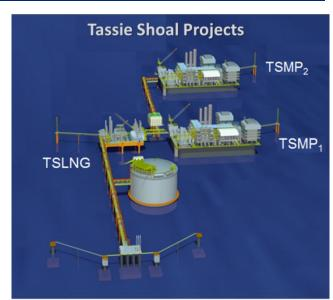
For each TSMP, feedgas of ~200 million standard cubic feet per day (Mscfd) is required, depending upon  $CO_2$  content, to enable the production of 5000 tonnes of methanol per day or 1.75million tonnes of methanol per annum. Tassie Shoal site is located adjacent to many undeveloped high  $CO_2$  gas resources in the region.
