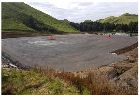
Figure 1 - Completed Pukatea drilling pad with existing Puka-1 and Puka-2 suspended wells protection zones visible
