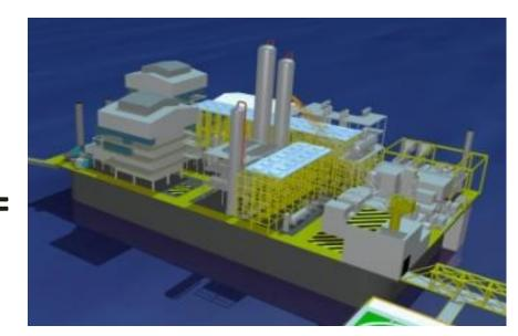
Methanol Plant on Concrete Gravity Structure (CGS)
