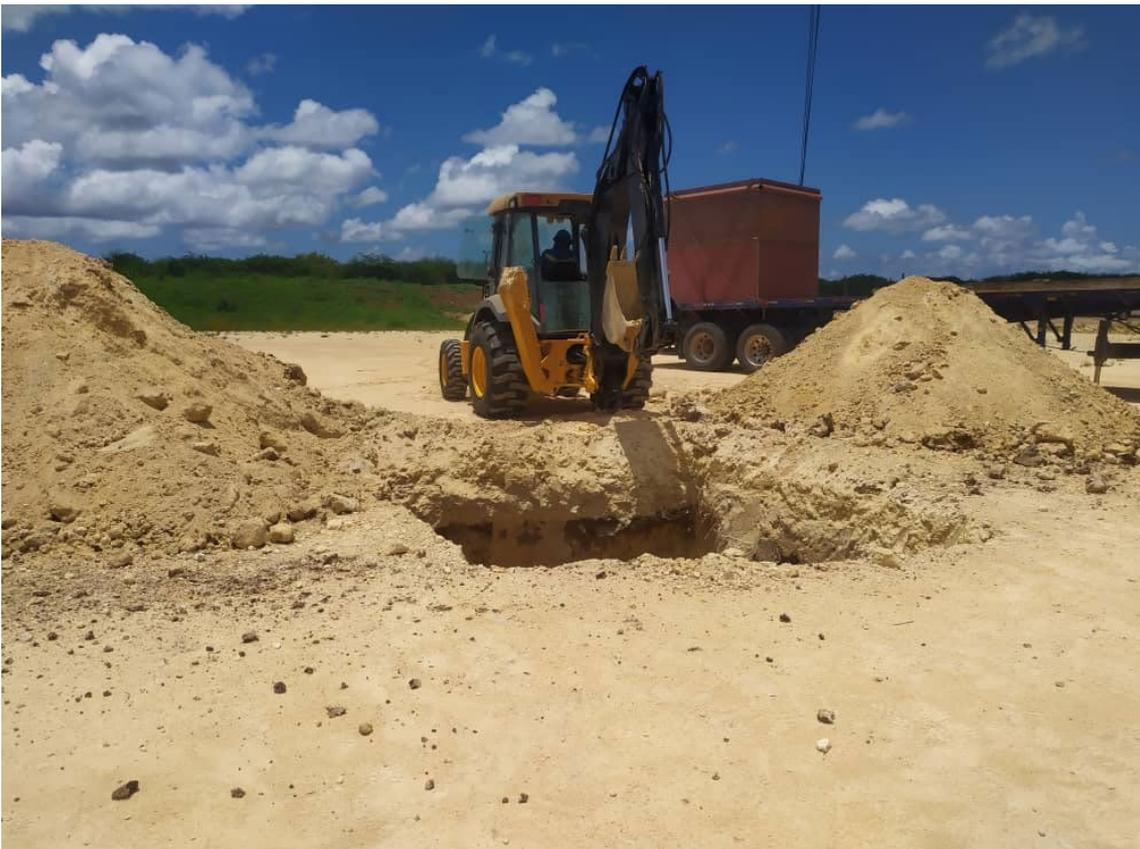
***Figure 2 - Construction of the cellar prior to the installation of the conductor***
