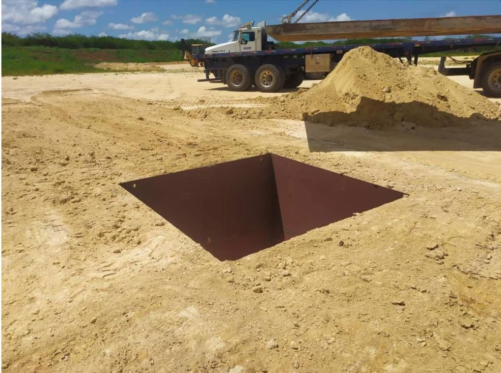
**Figure 3 – Completed cellar to provide structural foundation for the drill program**
