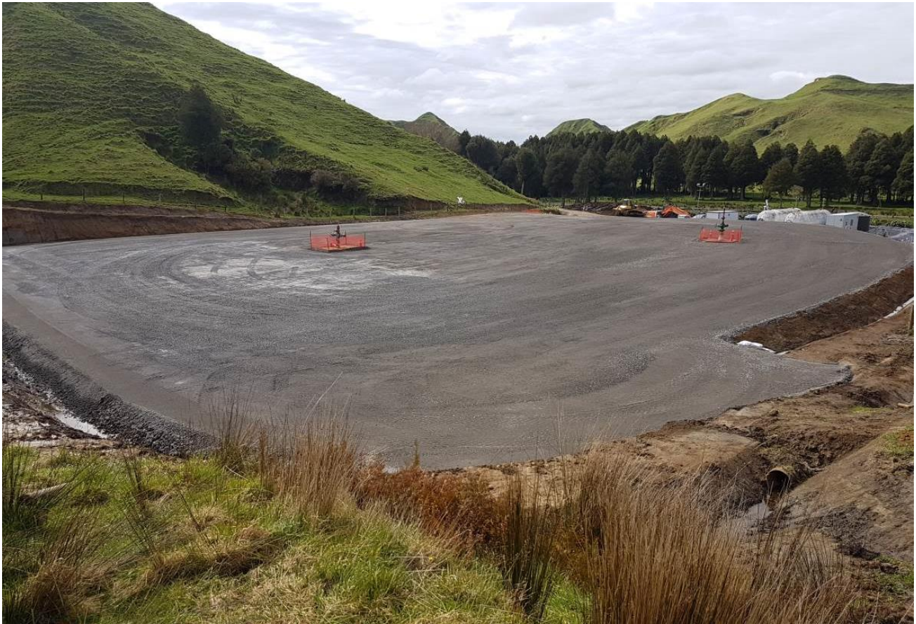
Figure 1 - Completed Pukatea drilling pad with existing Puka-1 and Puka-2 suspended wells protection zones visible
